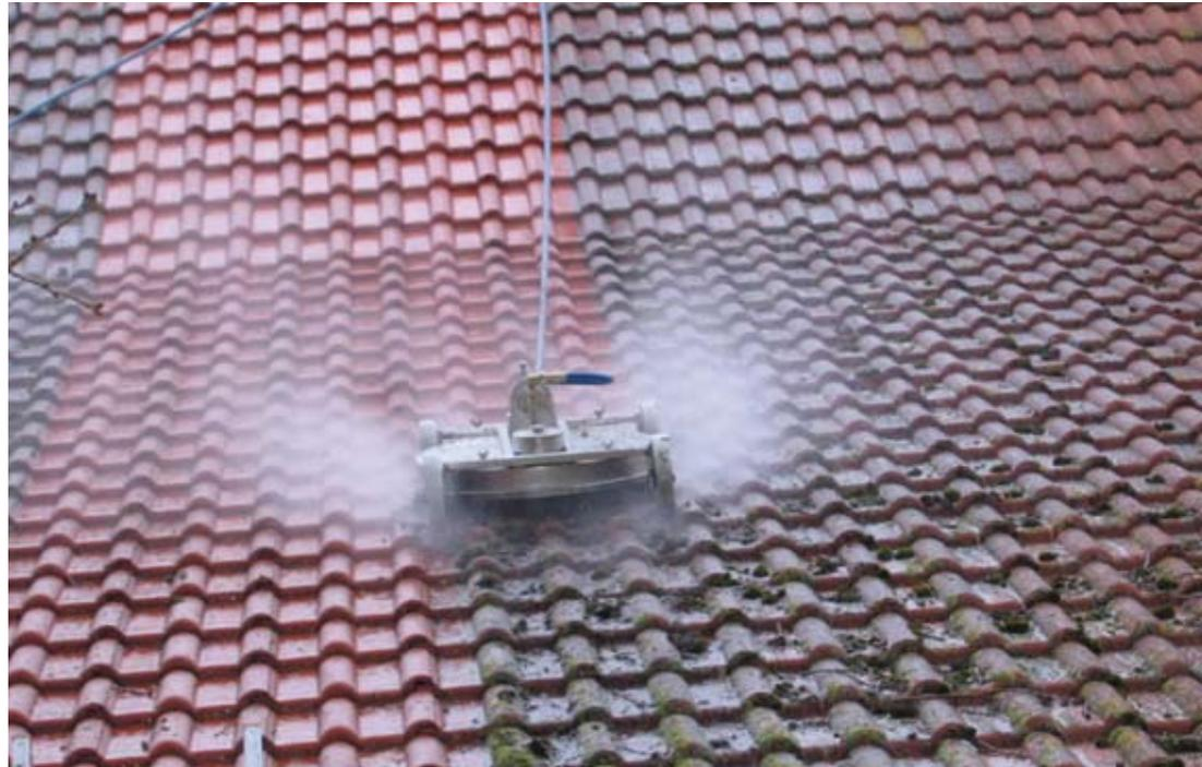
The Dynajet® roof cleaning system (DRS), here used on a heavily moss-covered concrete tile roof.
