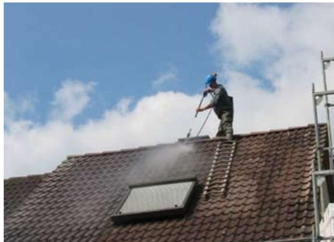
Conventional manual cleaning, with all its drawbacks and risks, can be reduced to a minimum.
