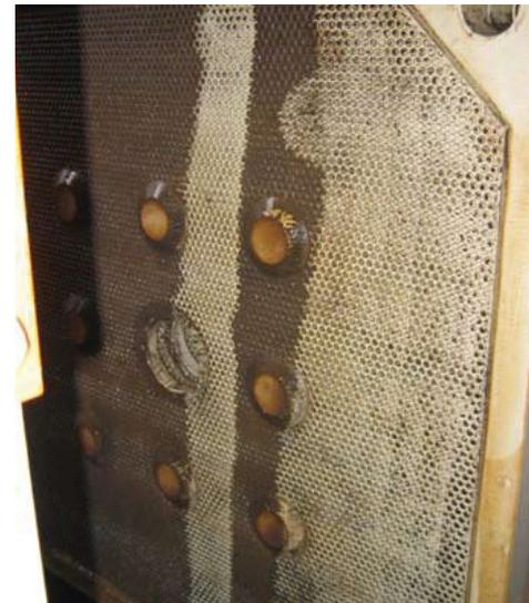
**Filter presses in sewage treatment plants are cleaned quickly and thoroughly with high-pressure. (here: Dynajet® 500<sup>me</sup>)**
