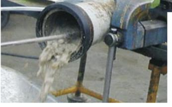
Tackling the concrete with an extended lance and a rotating nozzle.
