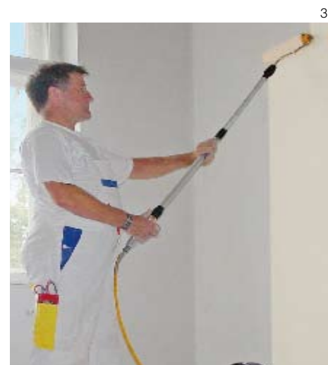
The roller is automatically supplied with paint from the airless device. The result is a perfect, completely even application of paint.
