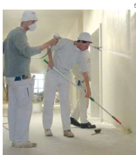
Whether inside or out, Putzmeister airless devices provide high quality paint application in the shortest time.
