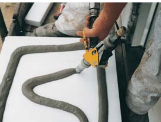
Our adhesives gun and the Sprayboy® make easy work of processing adhesive mortar for heat insulation composite systems.
