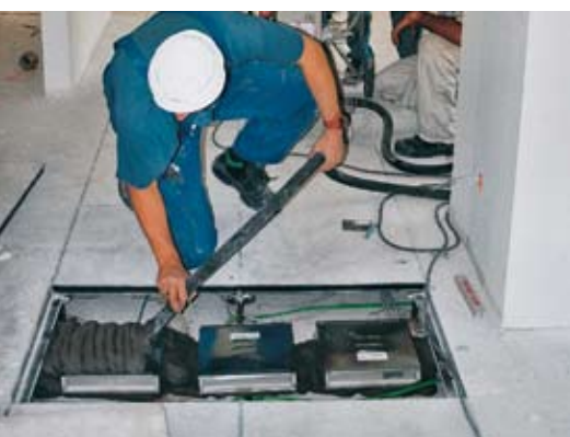
The issue of "fire protection" is becoming increasingly more important. Here distribution shafts are being sealed off.
