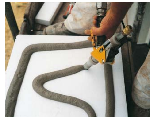
You can use the MP 22 without any problems for more sophisticated operation such as here for heat-insulating material.
