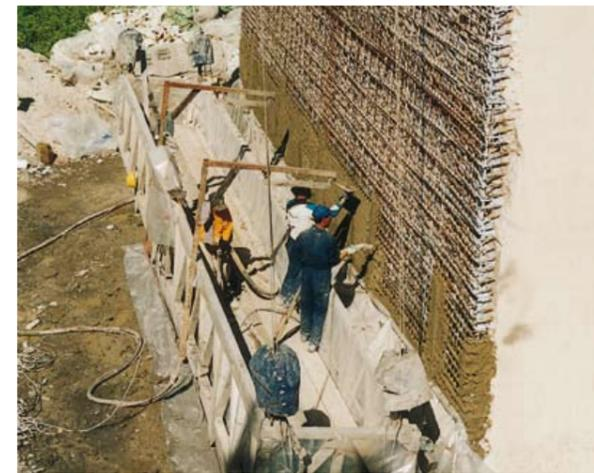
They are also extremely suitable for large jobs, as here for the concrete refurbishment of a motorway bridge in Italy.
