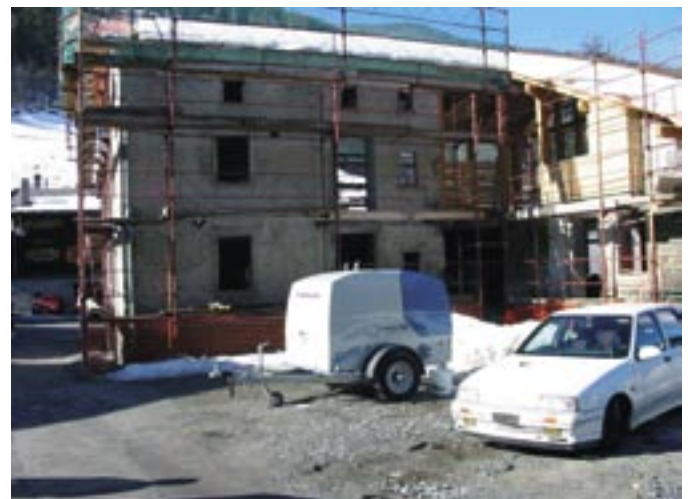
The historic museum had been plastered over in the course of time. Now one wished to return it to its original state with the natural stone masonry on show
