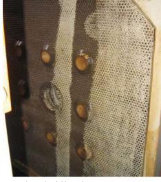
Filter presses in sewage treatment plants are cleaned quickly and thoroughly with high-pressure. (here: Dynajet® 500™)
