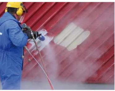
2,500 bar working pressure and cold water can remove even the most stubborn paint coatings.
