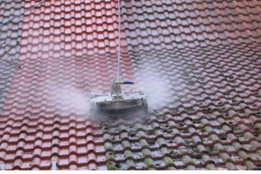
The Dynajet® roof cleaning system (DRS), here used on a heavily moss-covered concrete tile roof.
