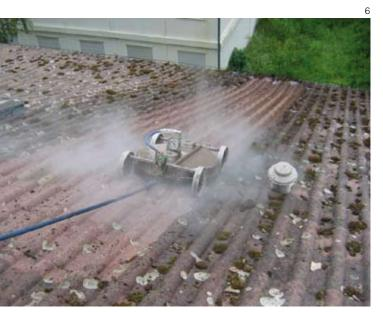
The DRS cleaning system can cover even large roof surfaces thoroughly, quickly and without having to walk on the roof.
