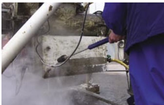
With hot water and rotating nozzle the cleaning results got even better.
