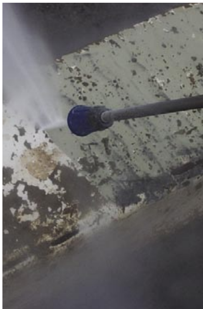
Here old paint stains are removed with a flat beam nozzle
